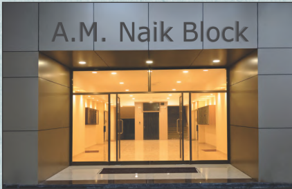
Newly Renovated A M Naik Block
