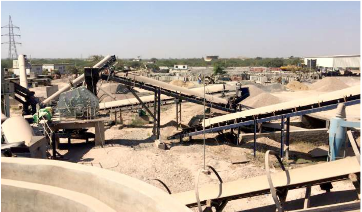
Figure 12. C&D Waste Processing Facility with 300 TPD Capacity, Surat
