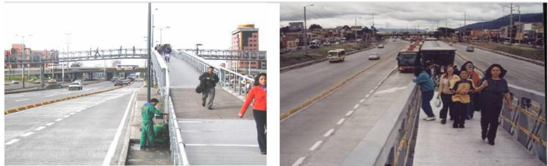
Figure 4.8 Grade separate crossings in Bogota
